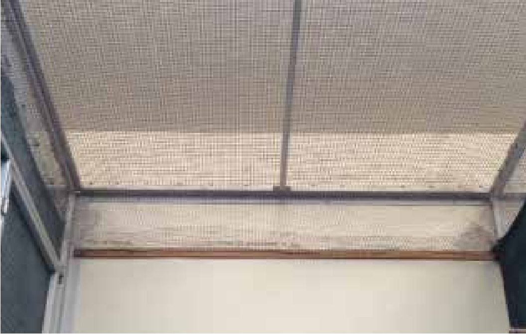
FIGURE 19: THE CEILING OF THE FLIGHT FITTED WITH A SOFT MESH TO PREVENT TRAUMA IF THE CHICK IS FLUSHED.PHOTO: JULIE MAHER©WCS
