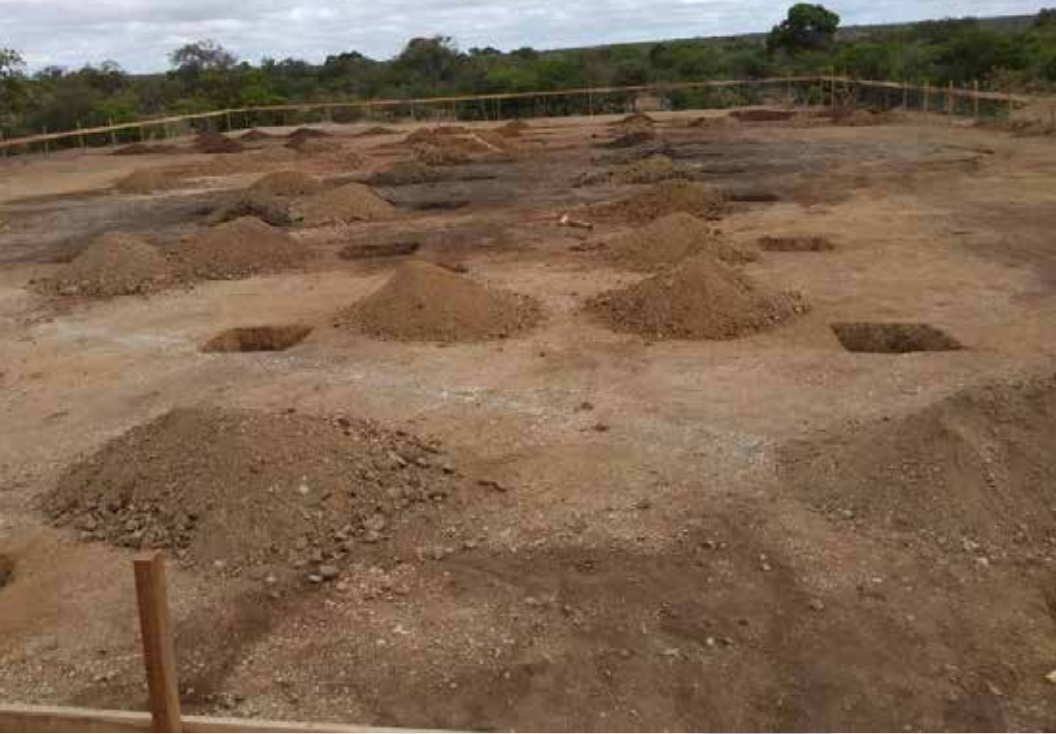
JANUARY 2019: LAND PREPARATION FOR BUILDING ACCOMODATIONS, RESEARCH AND VETERINARY FACILITIES
