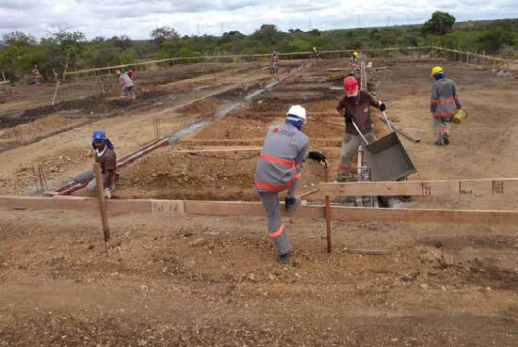
FEBRUARY 2019: STARTING OF THE RELEASE FACILITY
